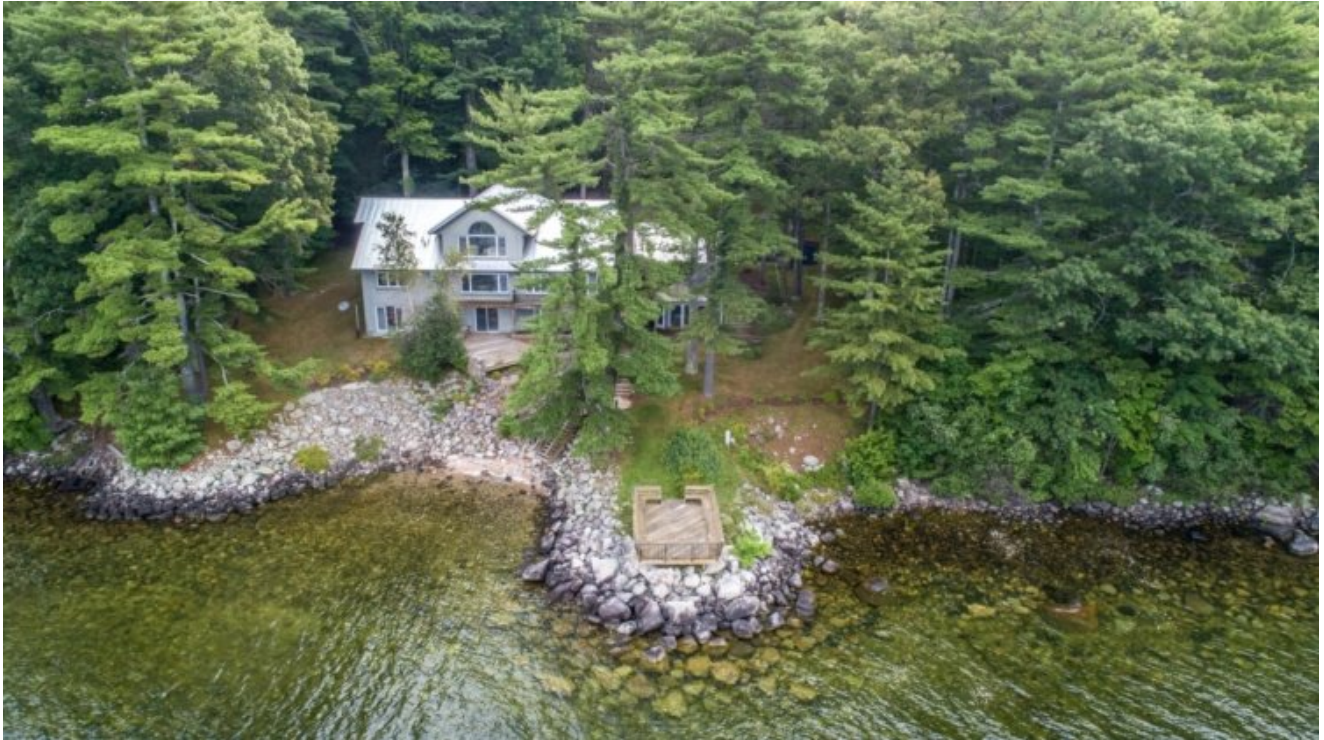
An August 2021 photo of the property at 28 Whitetail Lane before construction was performed. Town of Raymond photo
